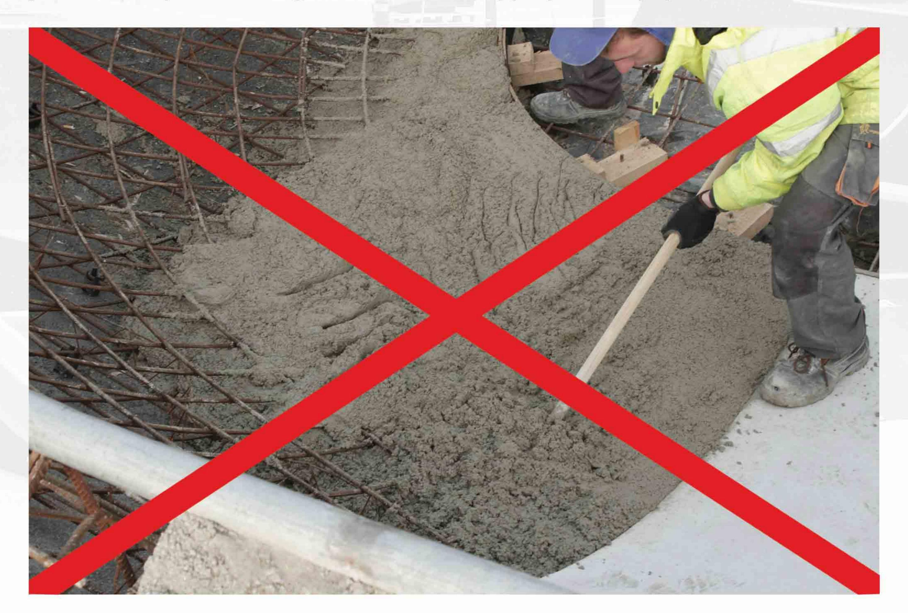
It is unacceptable to apply concrete by gravity - directly from a pump or shovel.
