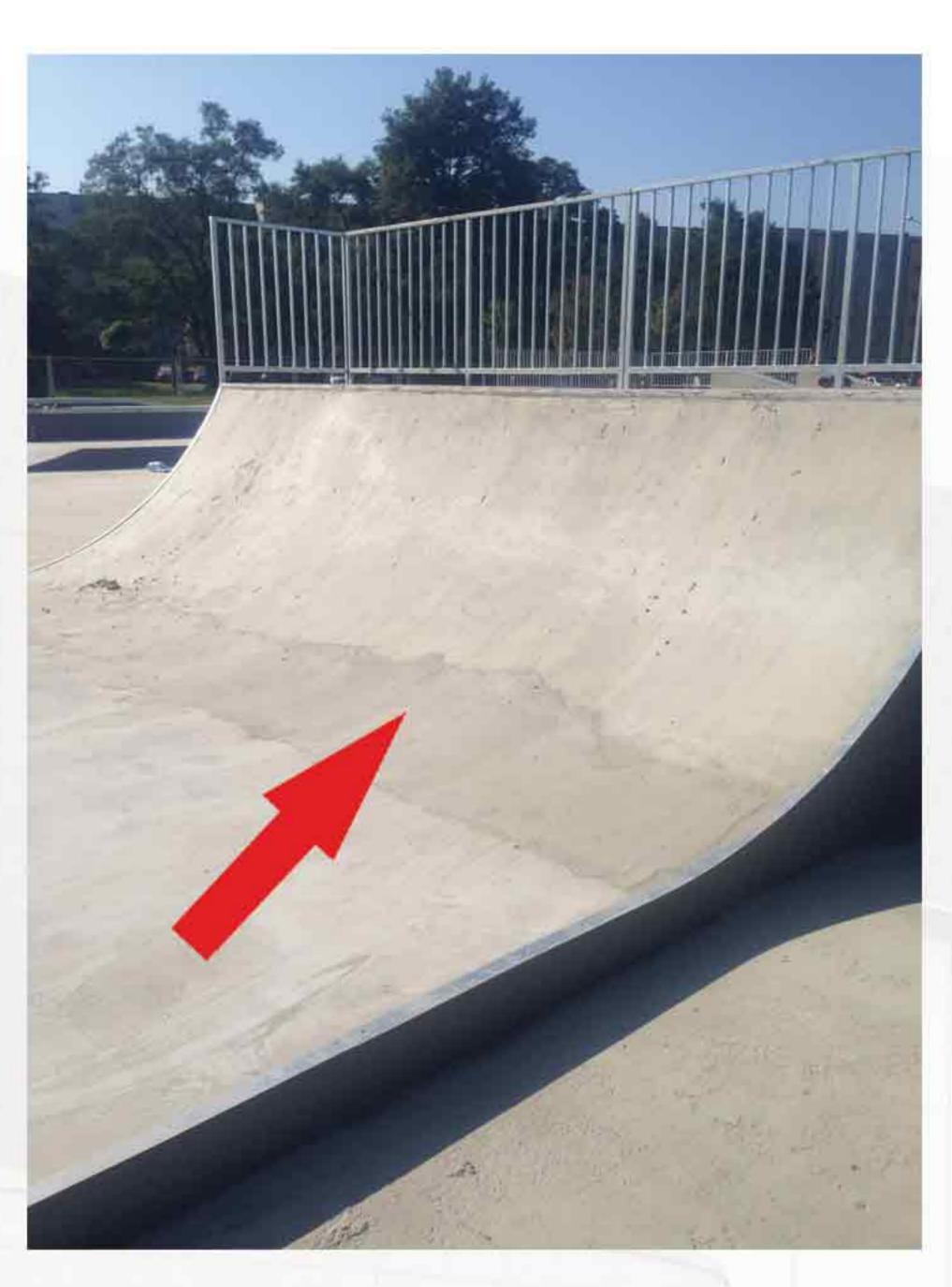
Device with poorly scuffed surface is unusable. Poorly scuffed device causes a large number of injuries to users and excessive wear of the equipment.
