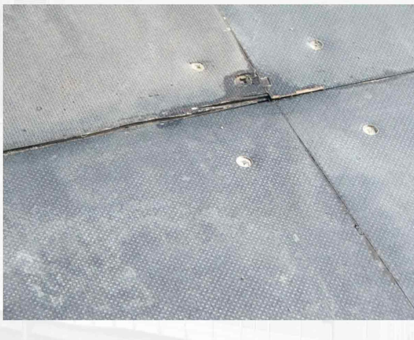
The use of inappropriate material causes rapid wear of the skatepark element and its riding surface, which directly affects the safety of users and the quality of driving.
