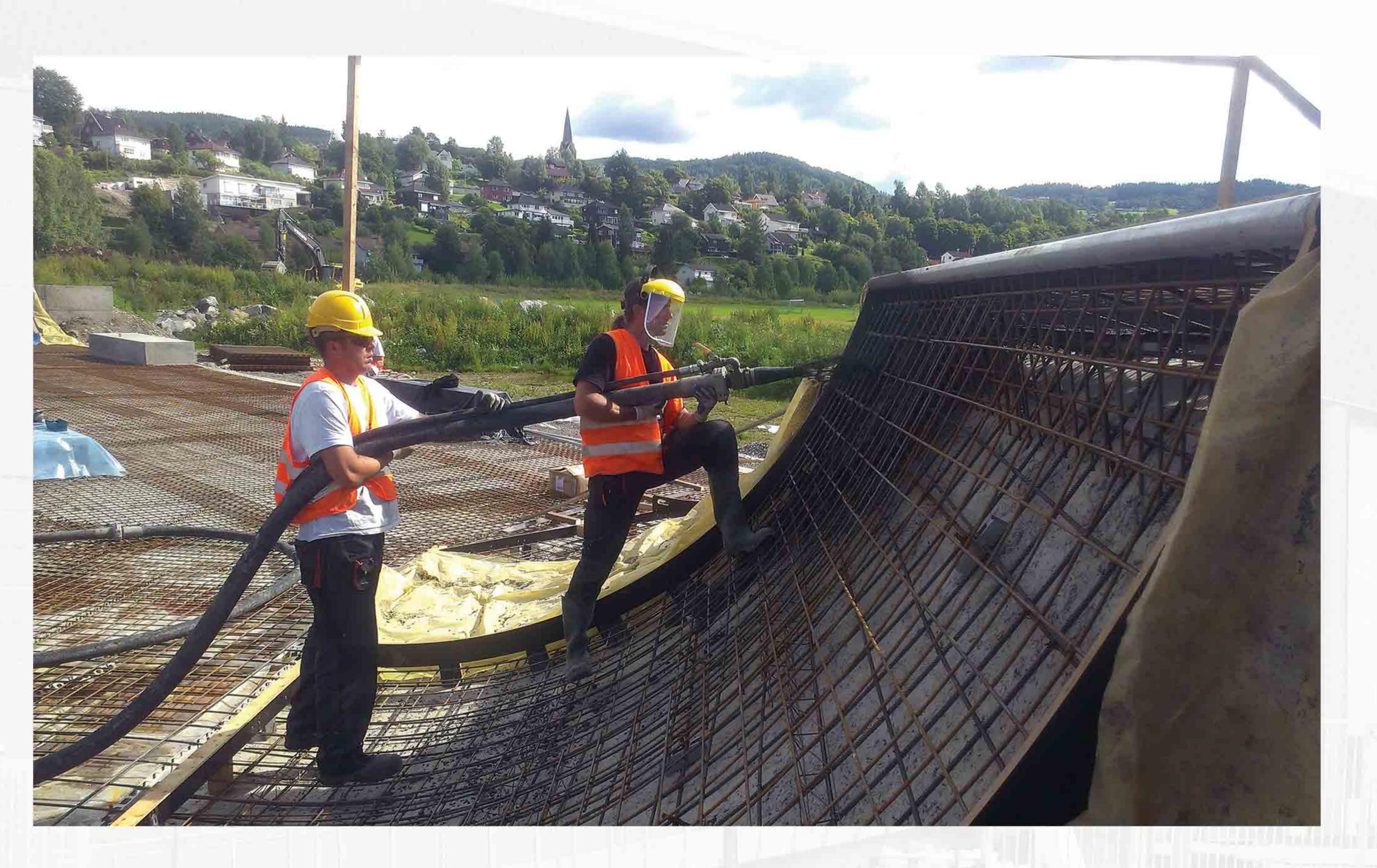
The application of concrete on curved and sloped obstacles should be performed by shotcreting with the use of appropriate equipment.
